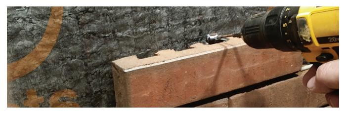
Our Dry-Stack mortarless option is a single 1-step installation. All you need is a brick, fastening clip, screw, butyl string, starter angle and rainscreen. With BRIKclad, you can begin enjoying your new clay brick wall in a matter of minutes!
